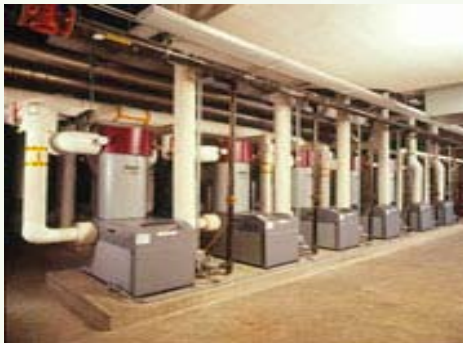
On larger applications condensing type water heaters can be used. They do not have the energy loss of maintaining hot water in a storage tank and they can operate at over 90 % energy efficiency. photo: Aerco Water Heaters
