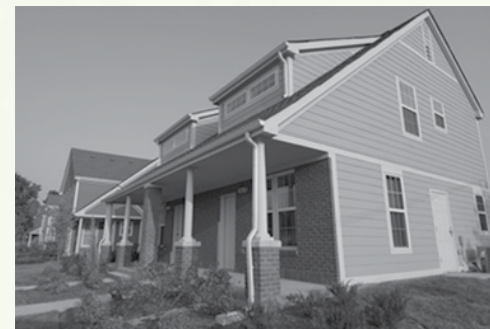
Sam Levy renovations included air sealing, higher R values in walls, attic & slab, new windows, and new HVAC system.
