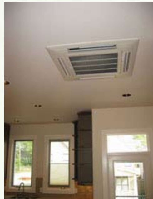
High efficiency, ductless split system air conditioning.
