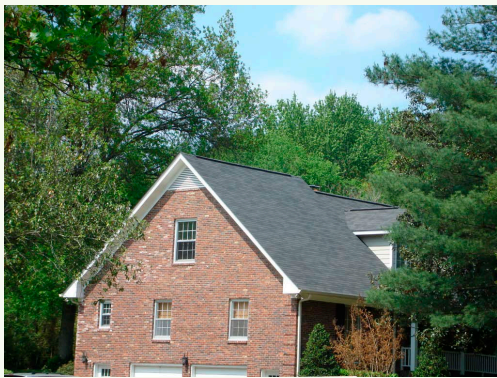
An example of a Solar Ready Home
